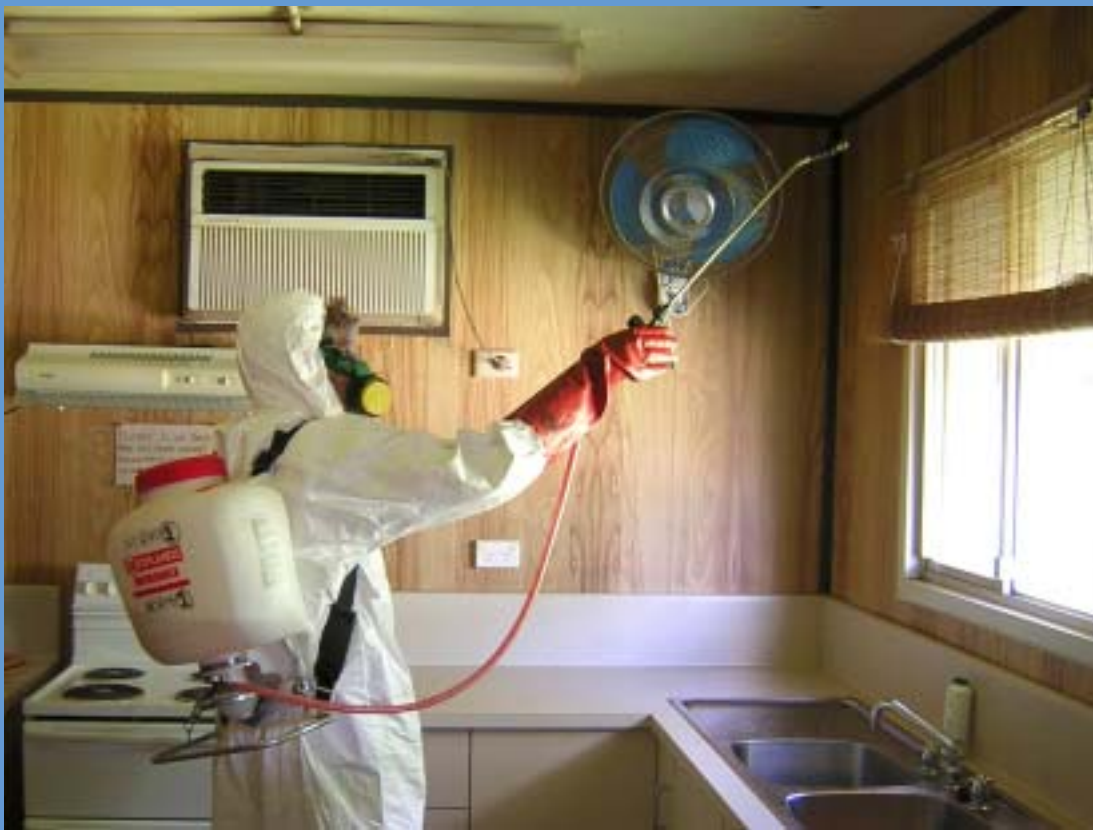
Fig 11: Careful planning and scheduling of work in homes is necessary so residents are not disrupted or harmed.
